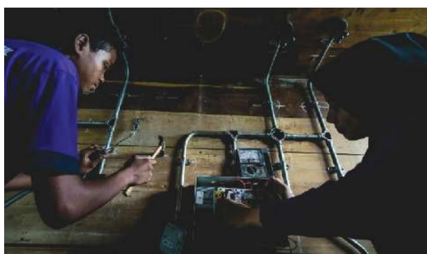
Picture 1: Electrical wiring installation is one of the semi-skilled courses offered in TVET programmes
